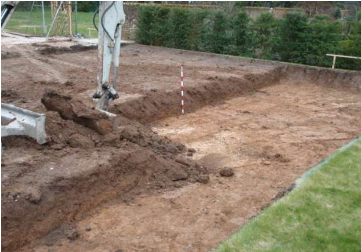
Plate 5. Excavation (looking south-east)
