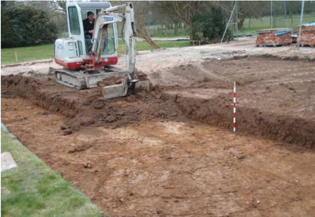
Plate 4. Excavation (Looking north-east )
